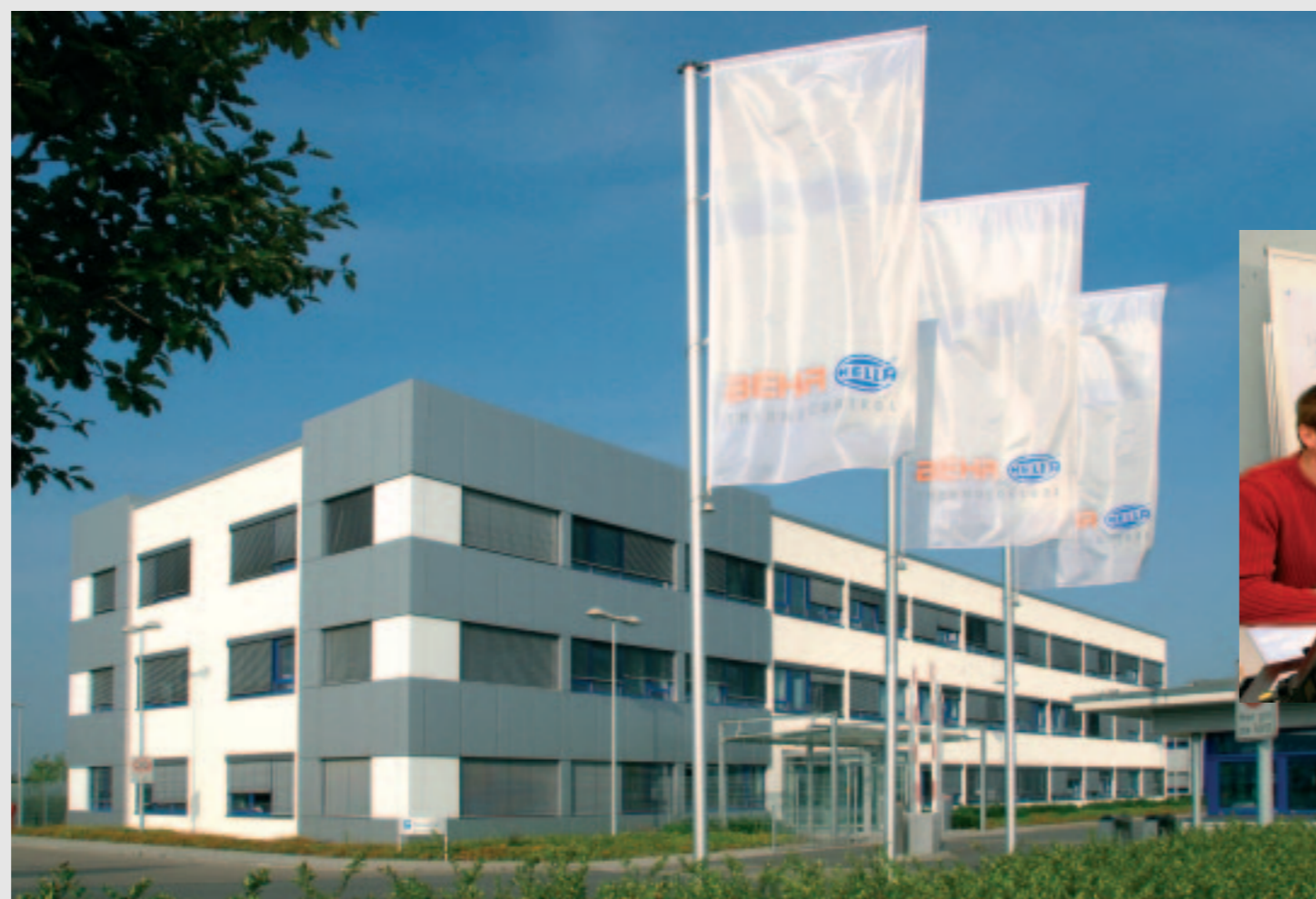
Innovation and transparency are not only demonstrated by the clearly structured architecture of the headquarters of Behr-Hella Thermocontrol in Lippstadt. They also form the solid basis of our company philosophy.
